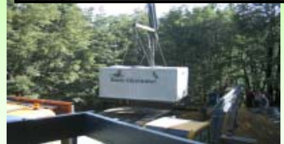
The septic tank is lowered into its hole.
