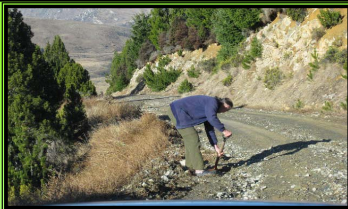
Roadman Ray at work on the cut-outs.
